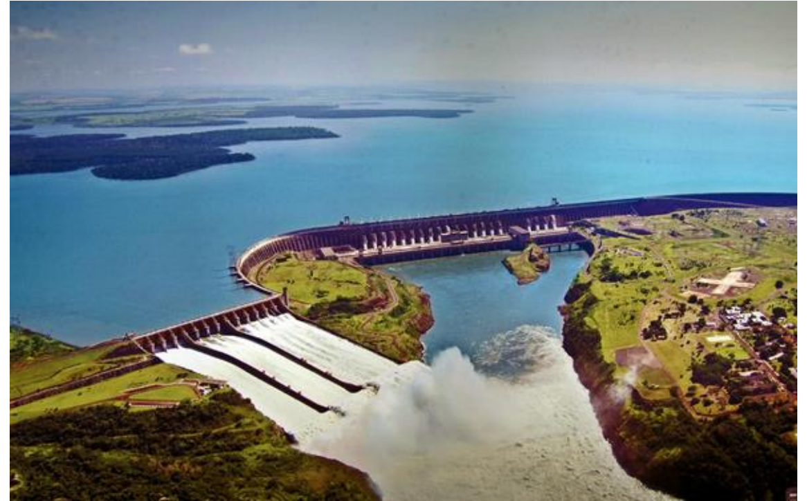
Itaipu Dam with Lake Itaipu in the background. Credit: Jonas de Carvalho
