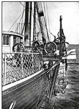
Invented in the late 19th century, the Sigsbee Sounding Machine was the first efficient piano wire sounding instrument. The basic design of ocean sounding instruments remained the same for the next 50 years. Image courtesy of the [NOAA Photo Library](#) (A new browser window will open.)
