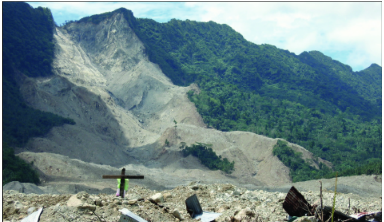
Debris from the February 17, 2006, landslide that buried Guinsaugon shows the effect of tectonic weakening. The landslide occurred along a fault line, where tectonic movement grinds and crushes the rock. This ground-up rock and soil on the mountainside had become more prone to landslides, especially after several days of rain. (Courtesy Stephen Evans)
