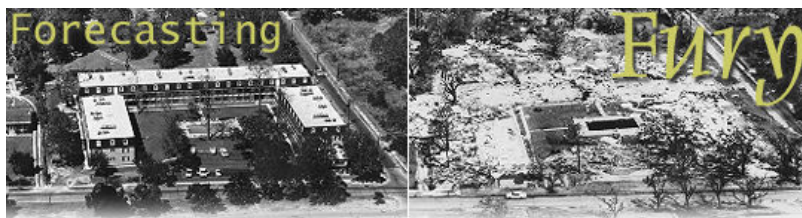
Apartments in Pass Christian, Mississippi, before and after Hurricane Camille (Courtesy of NOAA, photo by Chauncy T. Hinman)
